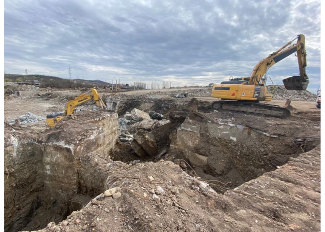
Demolition of existing coal power plant at RoPower's Doicești, Romania site
