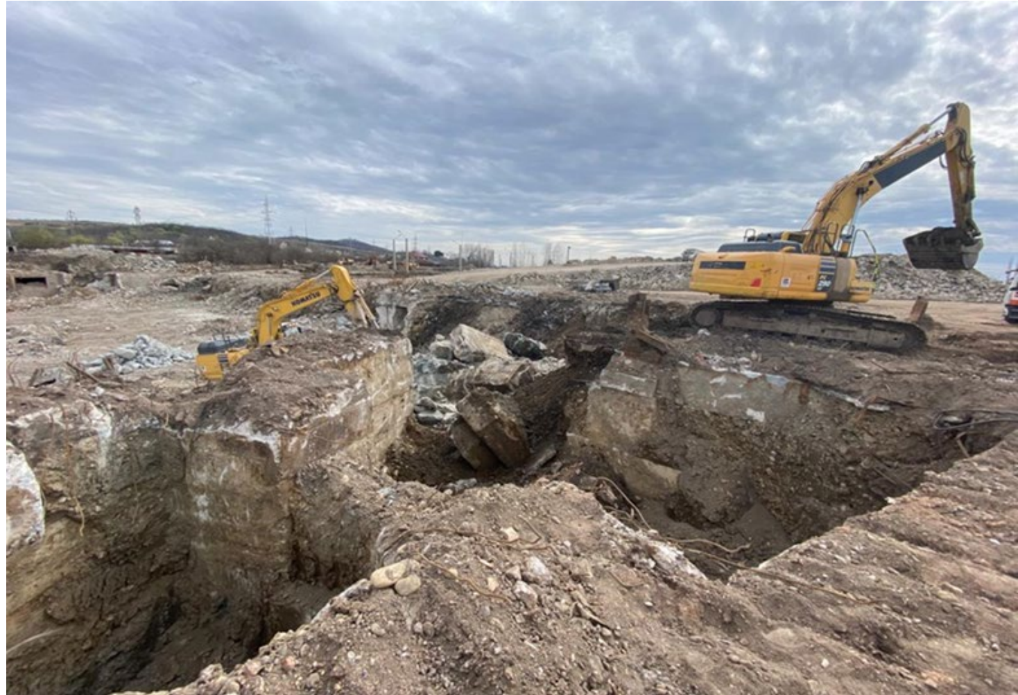
Site demolition of existing coal power plant at Doicesti, Dambovita
