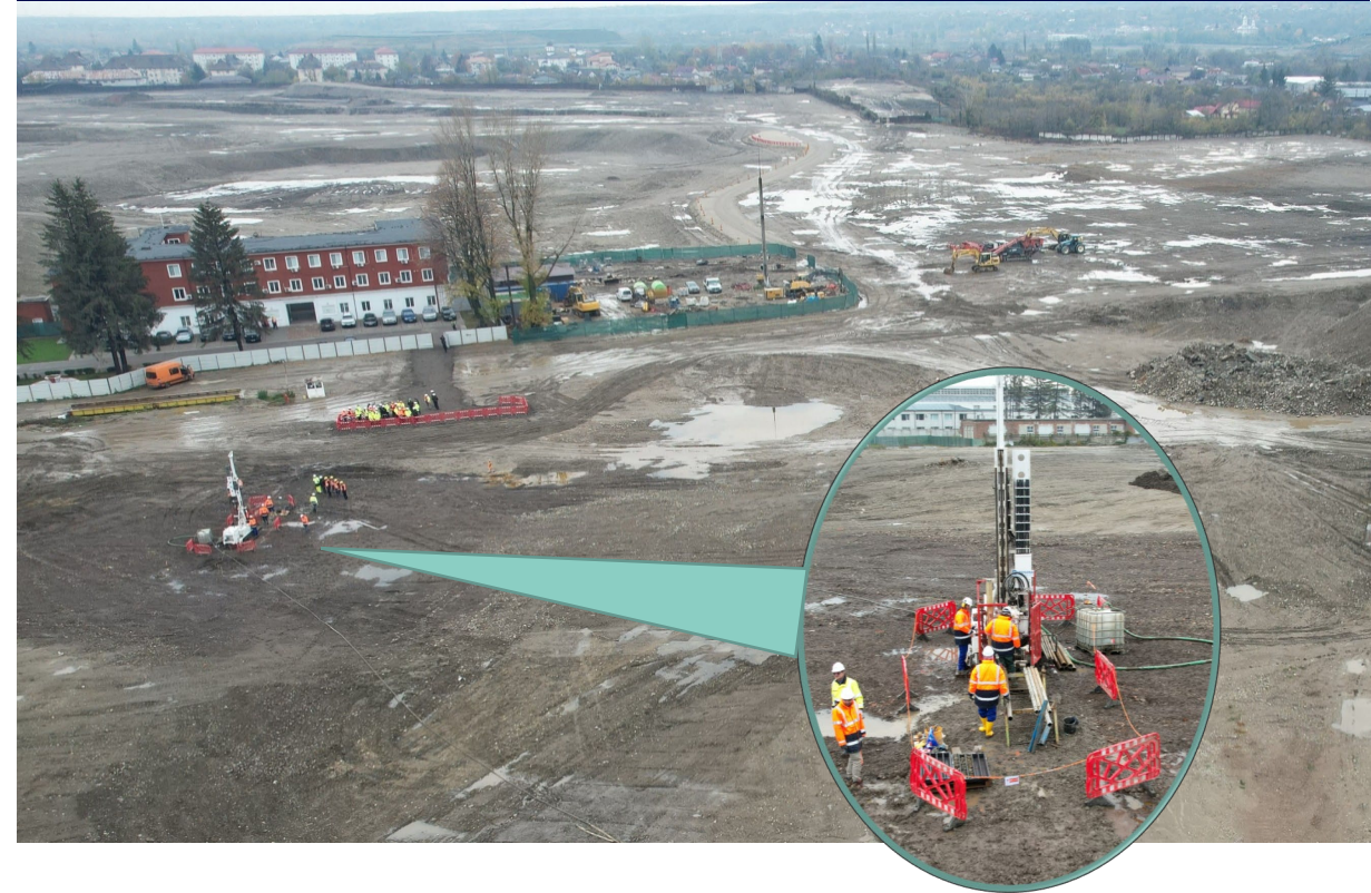
Aerial Shot of Future Site of RoPower Plant in Doicești, Romania; Drilling Cores to Characterize the Site for Seismology (1)
